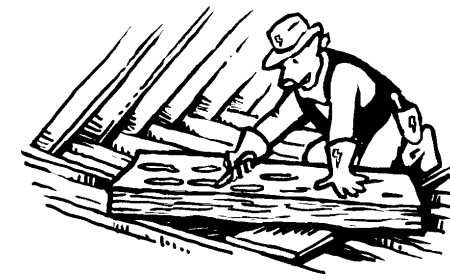
IF YOU INSTALL ADDITIONAL INSULATION, IT SHOULD BE UNFACED—OR USE A KNIFE TO FREELY SLASH THE VAPOR-BARRIER TYPE.
